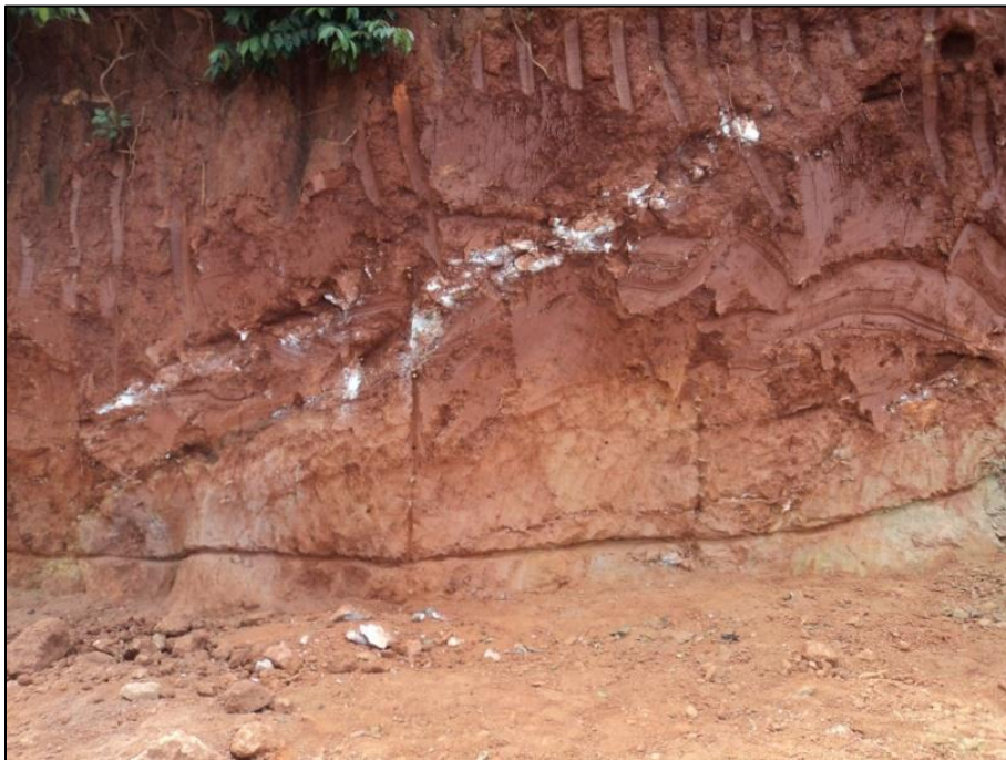
Figure 25 Road cutting showing horizontal and vertical channels from sampling.
